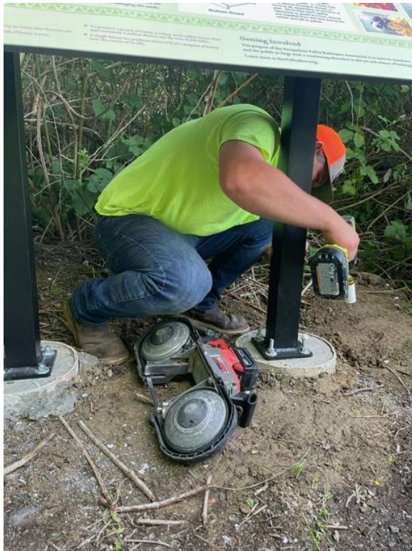
A specialist from Issaquah's FastSigns trims the extra bolts on one of the new signs. Juetten photo
